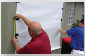
Quick and easy installation of the hurricane fabric with nylon hurricane clips
